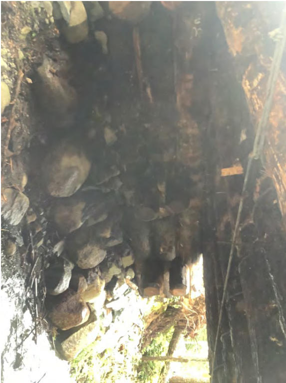
Left Bank Abutment when facing downstream
