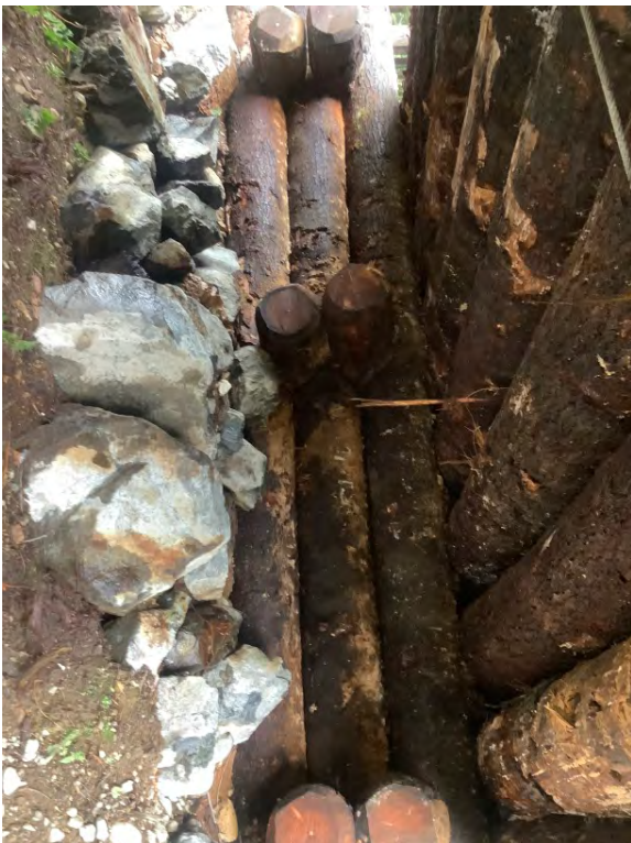
Right Bank Abutment when facing downstream
